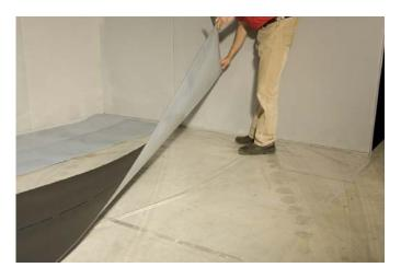
Turn over the Elastilon so that the smooth protective layer is on the upper side.
