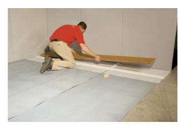
The first parquet section or board is now positioned on the spare film.
