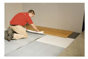
The second parquet section is pushed into the first until it locks tightly; following this, the spare film between Elastilon and the parquet boards is removed. From now on, work is carried out with the **actual** protective layer of Elastilon.
