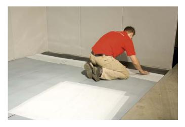
Fold back the protective foil of the adhesive layer over a width of one or two boards. The adhesive layer is now exposed.
