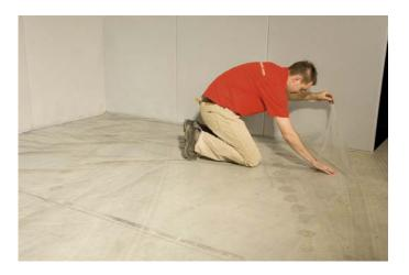
Place a polyethylene moisture barrier on the sub floor in strips with an overlap of 20 to 25 cm.
