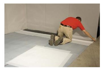
Carefully place the spare film onto the exposed adhesive layer with the fold facing the wall.
