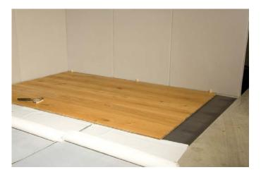
From here onwards, several rows can be positioned seamlessly before the protective layer between the wood and the Elastilon is removed.
