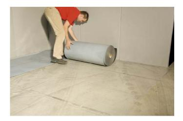
Roll out the Elastilon over the polyethylene moisture barrier in rows next to one another (the Elastilon strips must not overlap).
