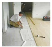
Elastilon is a strong elastic underlay that has an elastic one-sided adhesive layer. This specially formulated layer is protected by a plastic tear resistant foil. Parquet or solid wood should be installed square to the direction of the underlay, after which the protective plastic foil, that is between the wood and elastic underlay, can be pulled out. The wooden parts are now tightly and permanently joined to the underlay.
